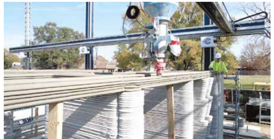
A construction worker watches as a 3-D printer lays concrete
