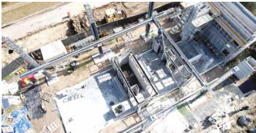
A 12-ton industrial 3-D printer is used to print concrete for the first 3-D-printed, two-story home under construction in Houston, Texas
